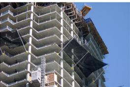
**Spider Sentry™ Perimeter Netting** provides perimeter fall protection for workers as well as debris containment for the environment below. Customizable panel configurations and various hardware mounting options ensure the Spider Sentry™ system can be engineered for virtually any structure or application.
