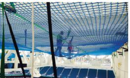
**Spider WorkWeb™** utilizes an engineered net and tension strap design to provide a unique and versatile work access solution at height, especially in locations where lifts and scaffolds are difficult to deploy. Predictable and easily navigable, the knotless construction of the WorkWeb™ netting improves the crew’s mobility and productivity while keeping them safe and secure.
