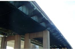
**Spider ContaiNet™** wraps around the debris source to prevent materials from becoming hazardous falling objects. Or when installed within 4 feet below a walking or working surface, ContaiNet™ also provides OSHA compliant fall prevention. Customizable with various strength ratings, liners and colors, each ContaiNet™ solution is fabricated to the exact job requirements for maximum safety and reliability.
